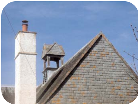
Bellcote, Old School, Steppingstone Lane
