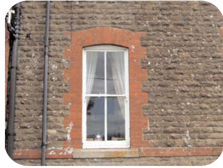
4-pane sash with brick dressings, The Old Vicarage
