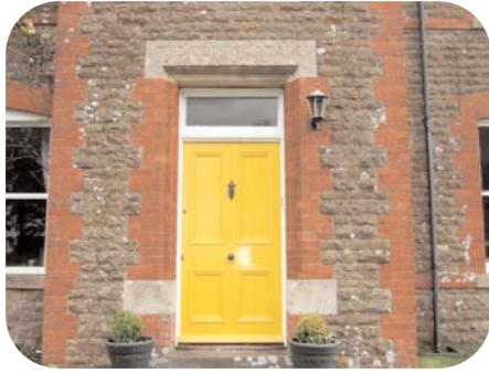
4-panelled door with overlight, The Old Vicarage
