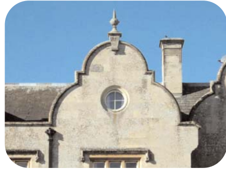
Oculus window, stone mullioned and transomed windows and finial
