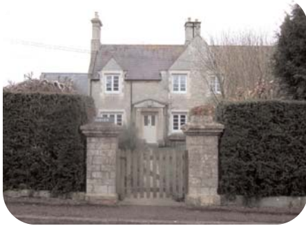
Chimney stack with moulded stone caps and bases, Fairview
