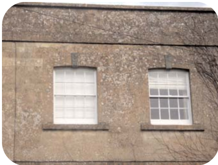
8/8 sash windows, Old Manor House
