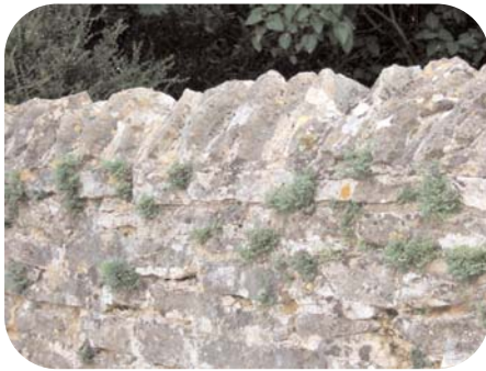
Stone wall with stone on edge of capping
